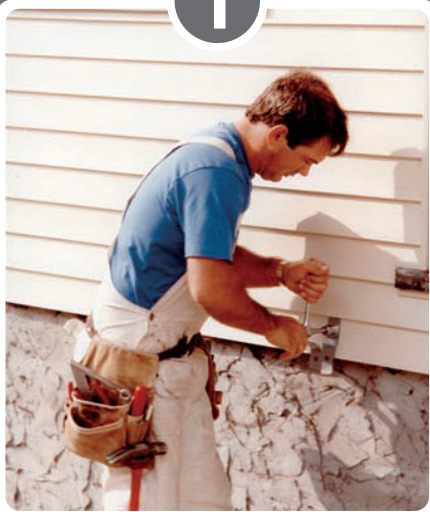
Install the Stratton Bracket®. Installez le Stratton Bracket MD .
