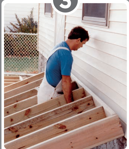
Set it into the brackets. l'installer sur les supports.
