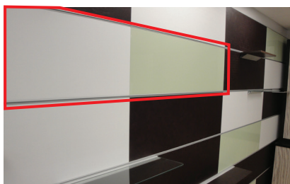
Snap in panels installed
