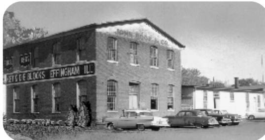
JOHN BOOS & CO. WOOD MANUFACTURING FACILITY EFFINGHAM, IL
