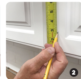
Measure from bottom of door to mark
