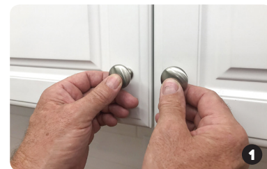
Place hardware (measure as needed) to find position you like; mark hole location
