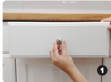
Place hardware (measure as needed) to find position you like; mark hole location (We are centering on width and height)
