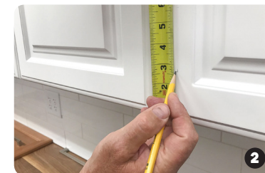
Measure from bottom of door to mark
