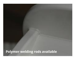
Because King StarBoard® ST sheet products are designed to resist water and grime, they cannot be painted and the use of adhesives is not recommended. If gluing is absolutely necessary, products such as 3M's Scotch-Weld DP-8005 and Lord Corporation's 7540-AB have been used with some success. Special welding rods, designed for use with polymer sheets, are also available.
