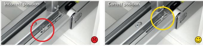
1.5 Are the screws tight? Are you using the correct screws?
