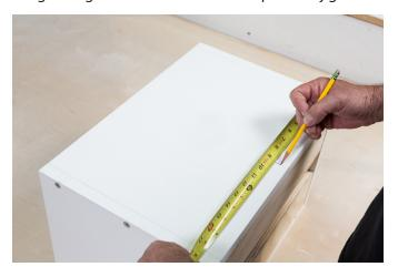
Slide jig along width of cabinet to align with pencil mark of desired puck light location.
