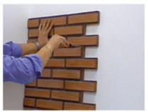
The previously joined screw and wall plug are inserted into the drilled hole and screwed until flush.
