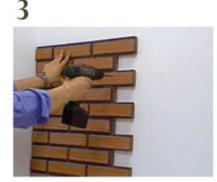
Position the panel on the wall and drill through the panel and wall, preferably in the cavities between the bricks
