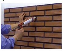
When the wall has been panelled, fill the joints and the drill holes with putty.
