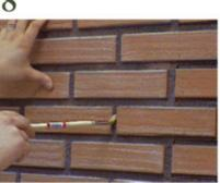
After filling the cavities with putty, smooth the joints with a fine paint brush.
