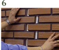
Fit, drill and screw all the panels covering the wall (No. 3, 4 and 5).
