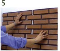
Fit the panels together. Due to their design, the insertion is perfect.
